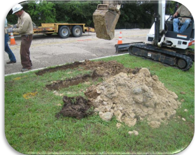
Confirmed both locations by excavation.
